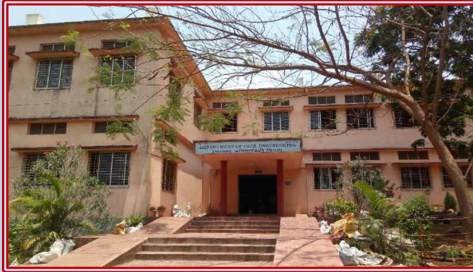
Front view of Civil Engineering Department, GIT (Lavel)
